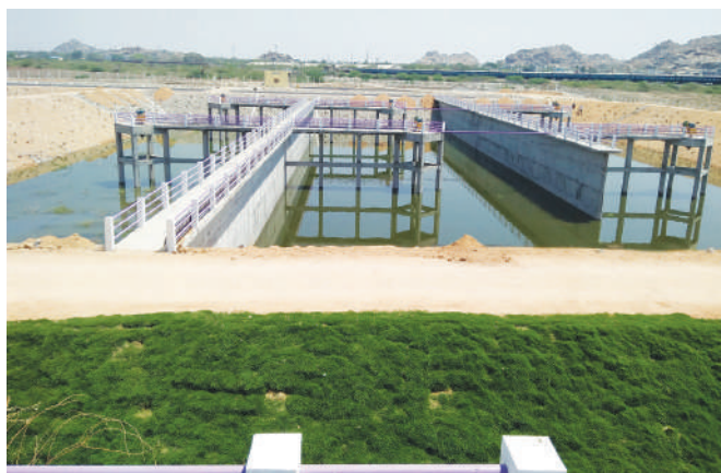
Sewage Treatment Plant at Raichur
