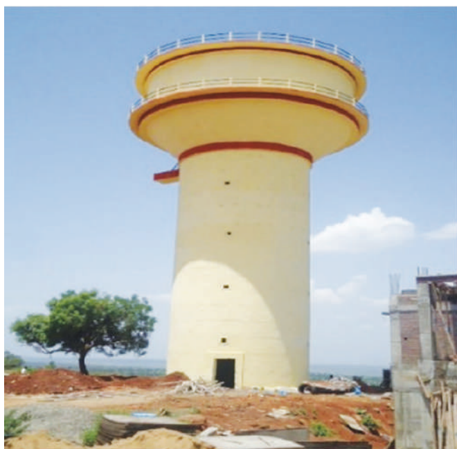
An Over Head Tank in Bagalkot
