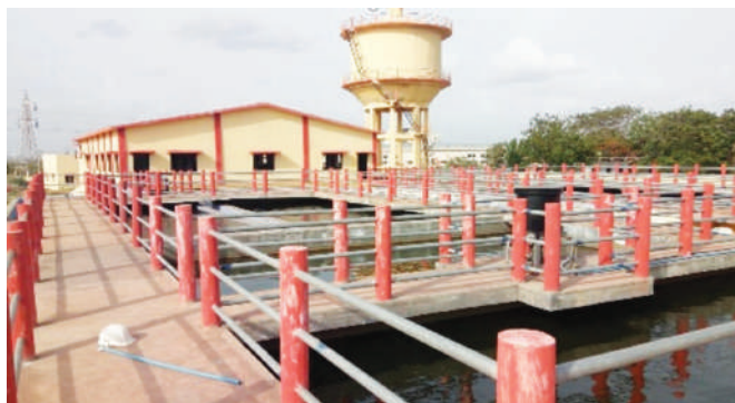
Water Treatment Plant at Ballari
